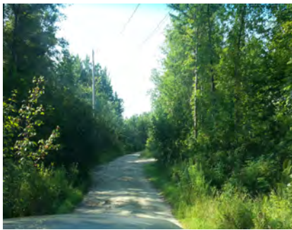
1. Condition of Existing ROW
