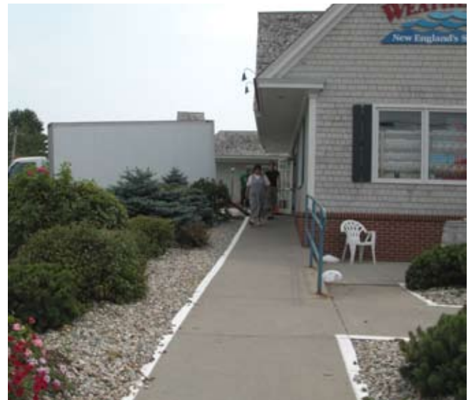
This round rock mulch may be an effective ground cover, but it can present a safety hazard when loose rocks end up in the walkway.
