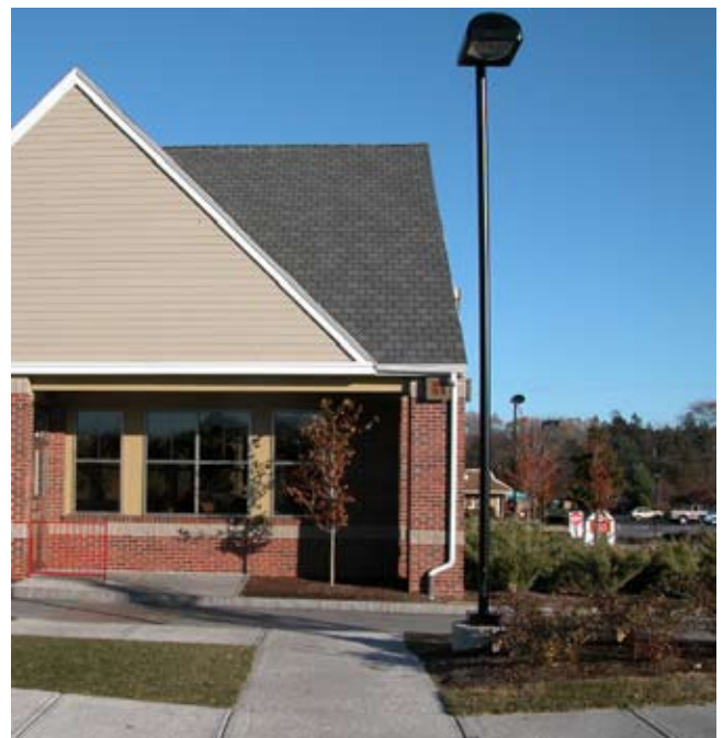
A cut-off fixture that complements the simple line of this commercial building. The fixture is mounted on an 18-foot pole on a one-foot base for an effective height of 19 feet.
