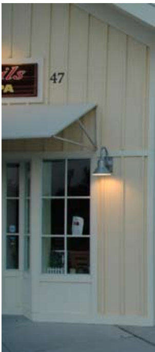
The wall-mounted light fixture on the right appears too small in relation to the height and scale of this large retail store. A proper installation is seen in the left photo.
