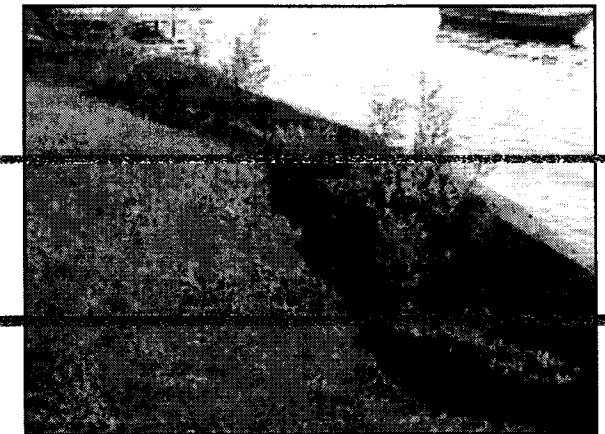
Once a "permit by rule" was obtained through the DEP, erosion control mulch and native vegetation were installed along the shoreline. This buffer strip will be able to more effectively slow the running stormwater, which will give it time to infiltrate into the ground.
