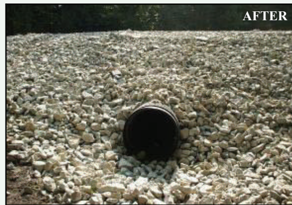
After: Riprap stabilizes bank
