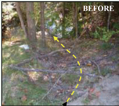
Before: Severe erosion. Large eroded gully above culvert outlet.
