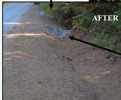
After: Turnouts installed to direct runoff into vegetation before the brook crossing. Shoulder & ditch stabilized.
