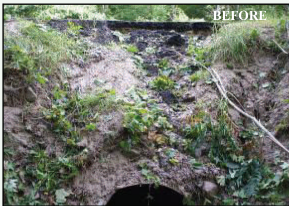
Before: Severe bank erosion
