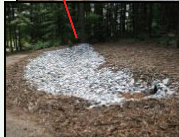
Sediment basin captures overflow of runoff from catch basins
