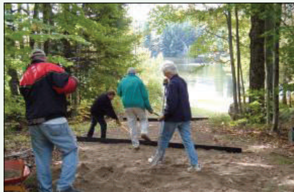
After: Rubber diverters direct runoff into stable vegetated areas and away from the lake
