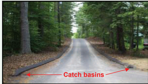
After: Curbing directs runoff into catch basins
