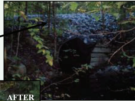
After: Turnouts installed to direct runoff into vegetation before the brook crossing. Shoulder & ditch stabilized.
