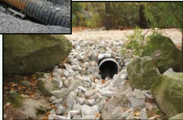
AFTER: Installed smooth bore polymer culvert. Stabilized inlet and outlet with stones (rip rap).
