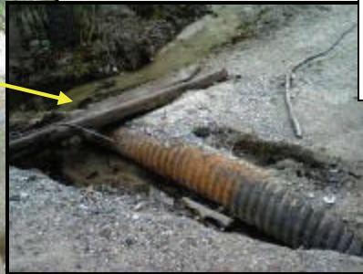
BEFORE: undersized, eroded culvert washed out in the Patriot's Day storm
