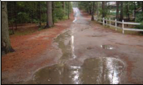
Before: Runoff erodes shoulder and private road with direct flow down eroded paths into the lake
