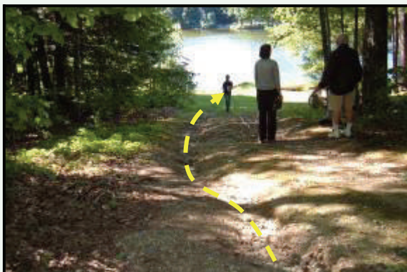
Before: Runoff causes eroded gully that washes sediment directly into Panther Pond
