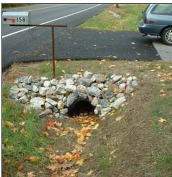
**Culverts**—Armor culvert inlets and outlets with rock riprap. Create 'plunge pools' to protect the outlet and trap sediment.
