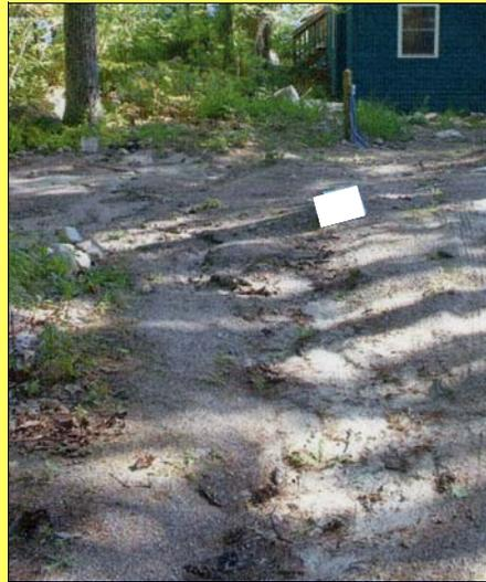
**Problem**—Water concentrates in ruts and erodes the surface of this driveway. A small basin at the base ponds water and traps some of the sediment.
