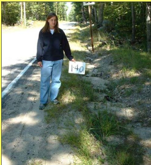
**Problem**—This site along Route 121 has moderate ditch and shoulder erosion and a large amount of winter sand that washes into one of the pond's feeder streams.
