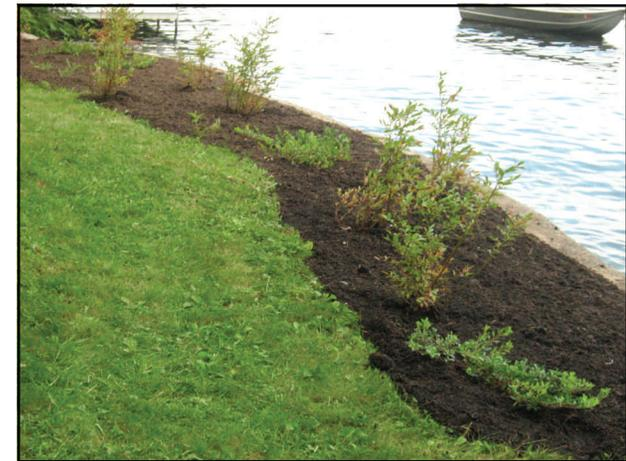
Once a “permit by rule” was obtained through the DEP, erosion control mulch and native vegetation were installed along the shoreline. This buffer strip will be able to more effectively slow the running stormwater, which will give it time to infiltrate into the ground.
