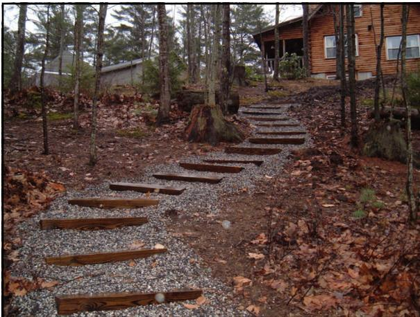
Infiltration steps and crushed stone were used to stabilize the eroding soil, as well as to allow stormwater runoff time to soak into the ground.
