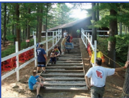
Camp Hinds—boy scouts convert gravel steps into infiltration steps to capture runoff washing down path
