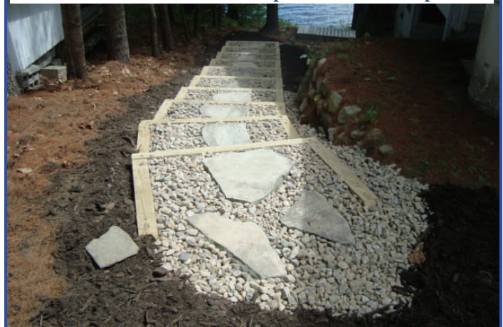
Crescent Lake - Infiltration steps installed on steep bank
