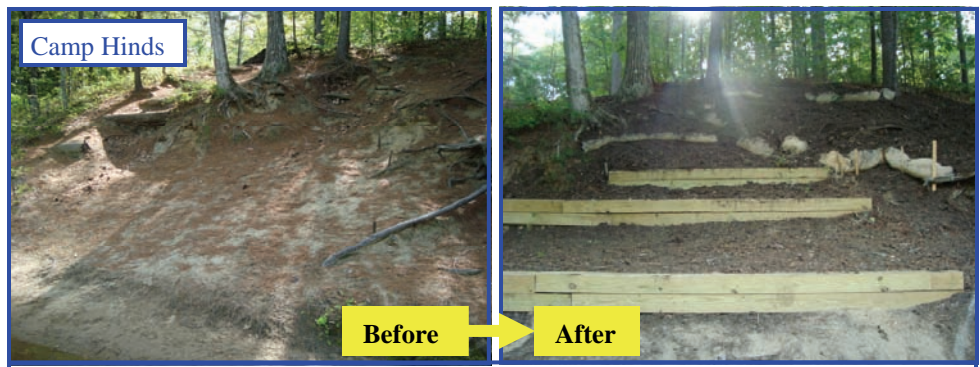
Before: Stormwater runoff and foot traffic erodes path and flows directly into the lake After: Waterbars, erosion control mulch and vegetation stabilize bank. Access limited.
