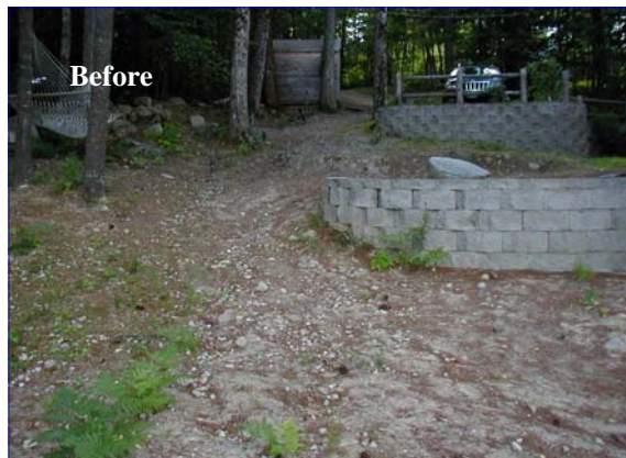
Moderate to severe erosion on steeply sloped side yard
