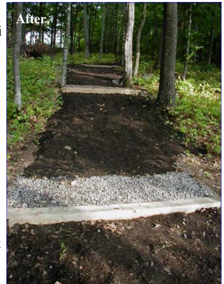
24 volunteers installed 2 open top culverts, 2 waterbars, and 7 timber stairs
