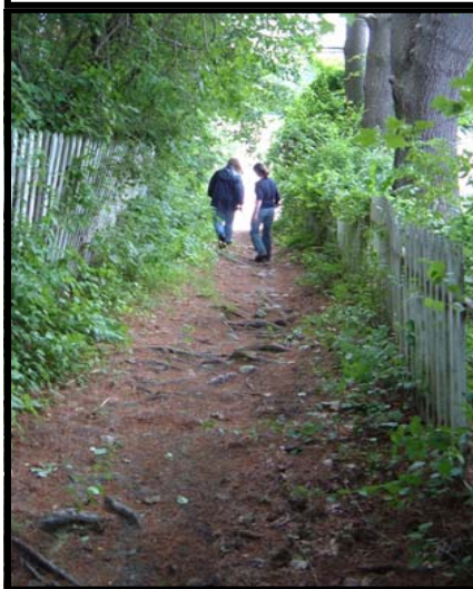
BEFORE: Chronic erosion on ROW with exposed roots and gully
