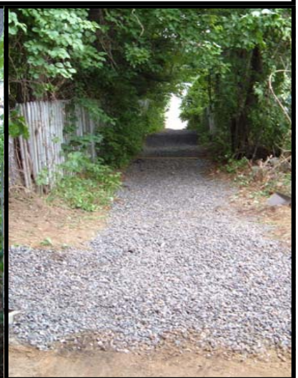
AFTER: Stone infiltration trench & path with waterbars
