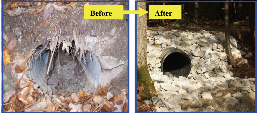
River Road Before: Culvert bottom rusted out, eroding unstable in/outlet After: Replaced culvert, rip rap in/outlet with rip rap (stone)
