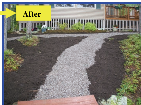
Before: Eroded & Undefined Path to Lake, Sparsely Vegetated Open Area After: Defined Crushed Rock Path, Erosion Control Mulch on Path Edge
