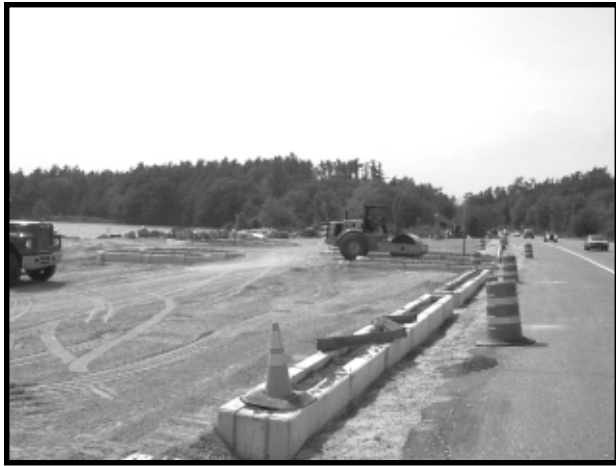
Raymond Beach Area Under Construction
