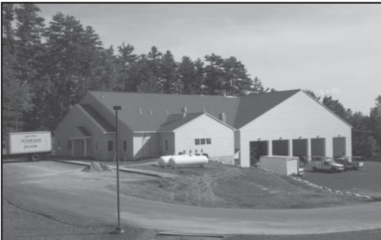
The new fire station nears completion.
