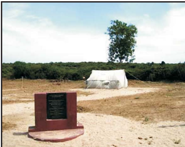
A view of the foundation stone with a temporary work tent and a single tree standing tall in the midst of the shrub jungle
