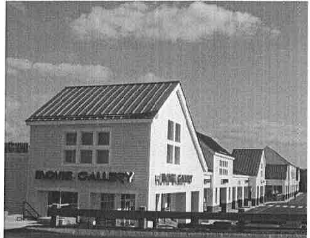
This smaller retail store attached to a large grocery has been designed as an individual building, with a separate entrance and architectural detailing. A covered walkway connects all the storefronts.
