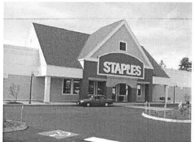
A similar building with a facade composed of New England forms and materials. The overhang provides protection for pedestrians and emphasizes the entranceway. The sign is overscaled (i.e., too large) for the facade.
