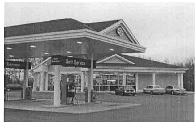
Lighting should be considered as an integral part of the canopy design. These canopy fixtures are recessed so the light source is not visible and do not create 'hot spots' that are distracting to the passing motorist.
