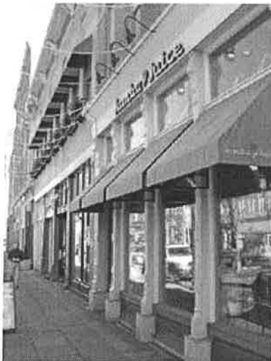
The awnings on this village building provide shelter for the window-shopper and add scale to the building.
