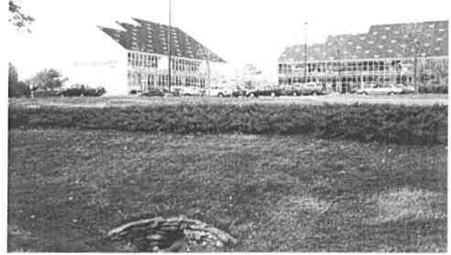
Motorists driving past this shopping center only see the low juniper hedge, unaware of the detention basin on the far side. Hand-placed stonework protects the end of the culvert.
