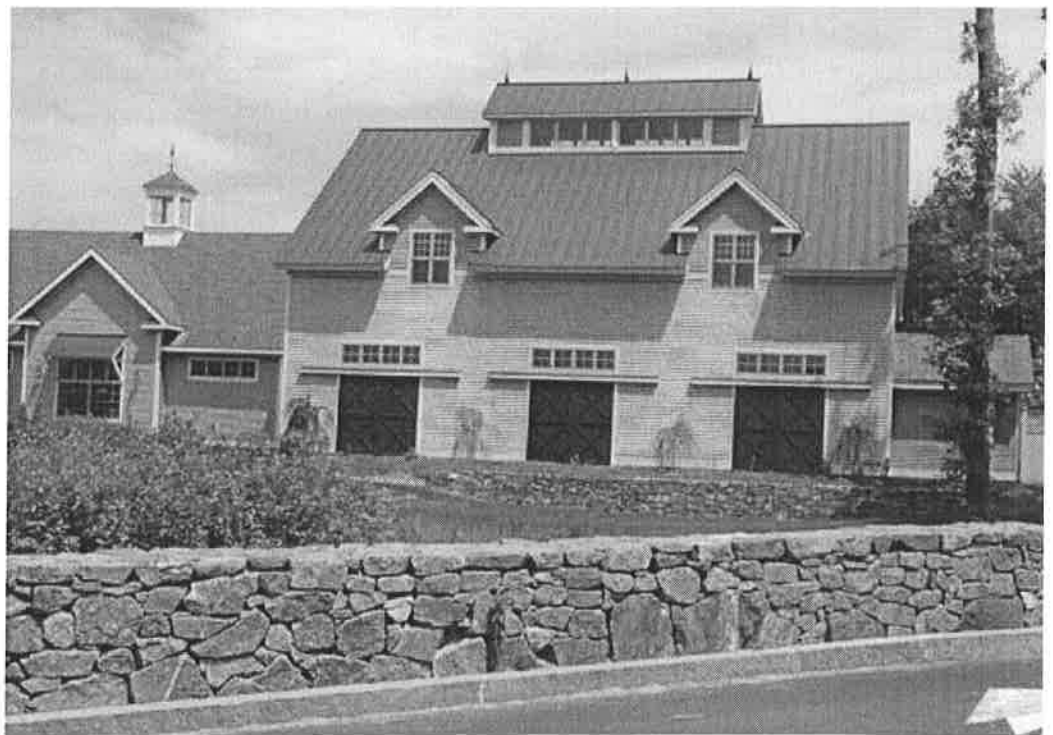
The scale of this large retail building has been reduced through variations in its roof line and roof materials.
