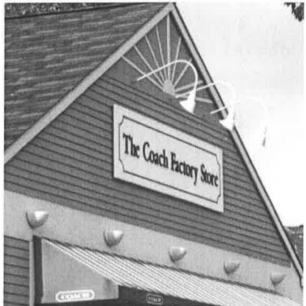
In both examples, the top-mounted light fixtures are well-located, aimed, and shielded so that only the sign is lit. The lighting fixtures compliment the signs and the buildings.
