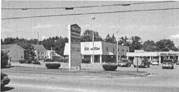
Typical commercial development lacking in scale, landscaping and pedestrian amenity. Parking lots are dominant visual elements.
