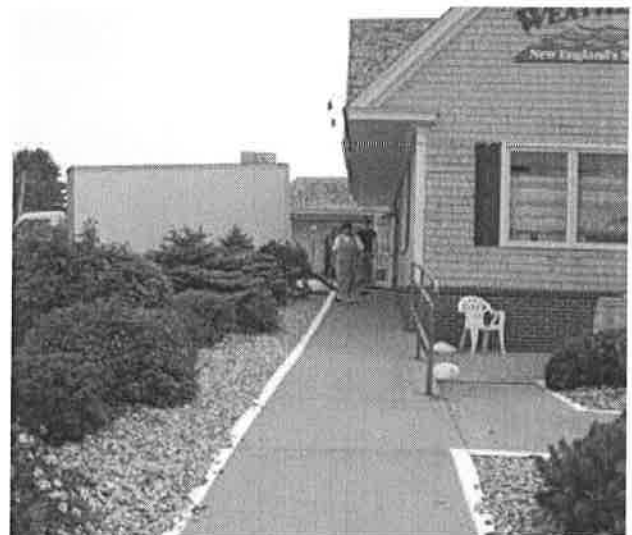
This round rock mulch may be an effective ground cover, but it can present a safety hazard when loose rocks end up in the walkway.
