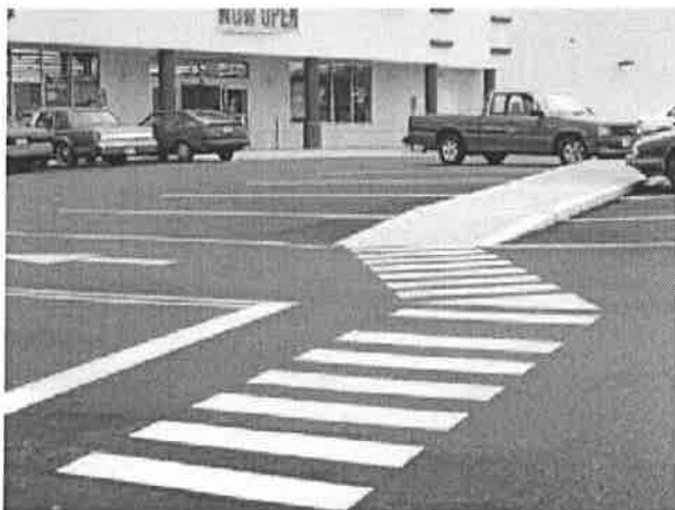
A raised walkway that provides a high level of contrast with the surrounding parking lot. However, the width of the walk is compromised by the overhang of the cars, making pedestrian movement difficult.
