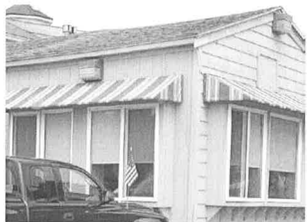
Unshielded facade-mounted lights are not allowed because they cause glare and spill light onto adjacent properties.
