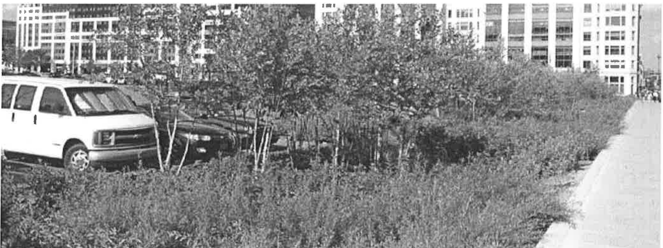
An infiltration area next to a parking lot provides an attractive and functional way to deal with on-site stormwater.
