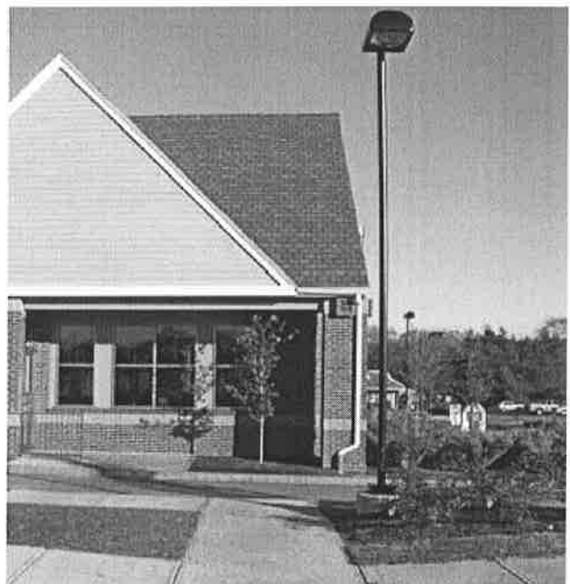
A cut-off fixture that complements the simple line of this commercial building. The fixture is mounted on an 18-foot pole on a one-foot base for an effective height of 19 feet.
