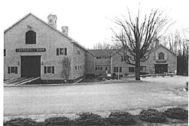
Drawing from traditional forms, the scale of this new commercial building has been effectively reduced by variations in the massing, wall projections, and careful attention to detailing.
