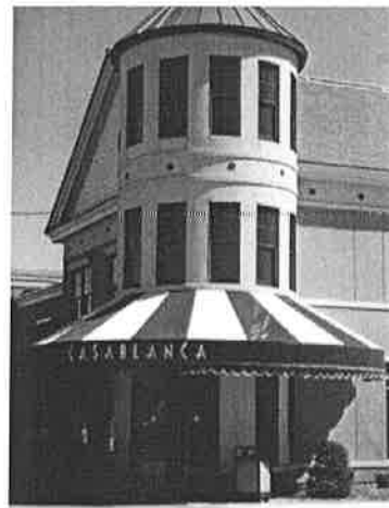
Canopies over doorways can emphasize the main entrance and provide effective protection from the elements. The name of the theater is incorporated into canopy and counted toward the total signage area.
