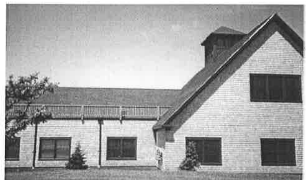
Roof-mounted mechanical equipment has been effectively screened by balustrades.
