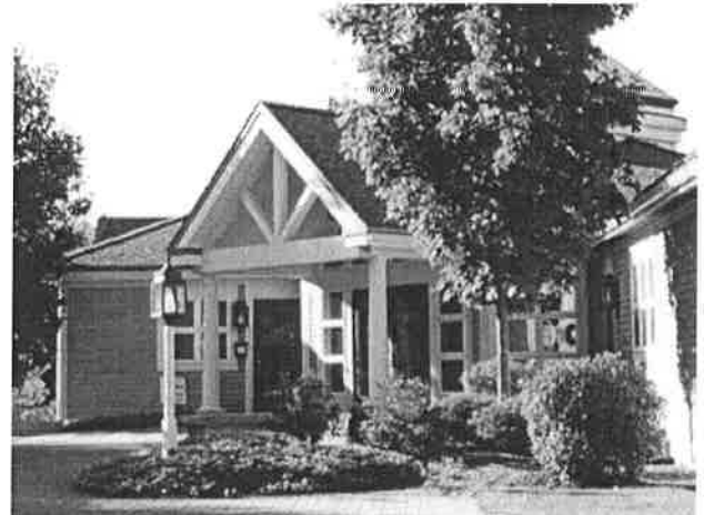
An informal grouping of trees, shrubs, groundcovers, and trees emphasize the front entrance of this office building.
