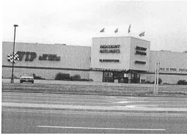
A flat roofed building that is designed as a large billboard with no variations in form to add human scale.
