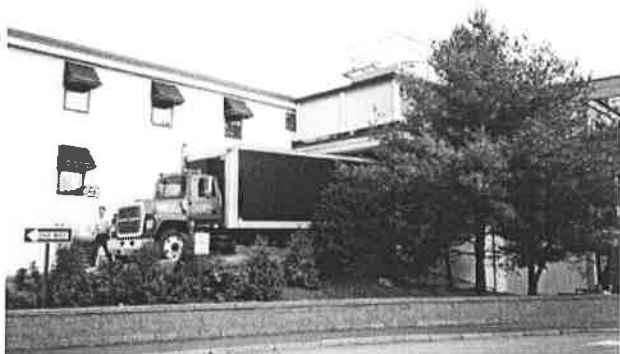
This service area is effectively integrated into the side of the building and well screened by an evergreen buffer.
