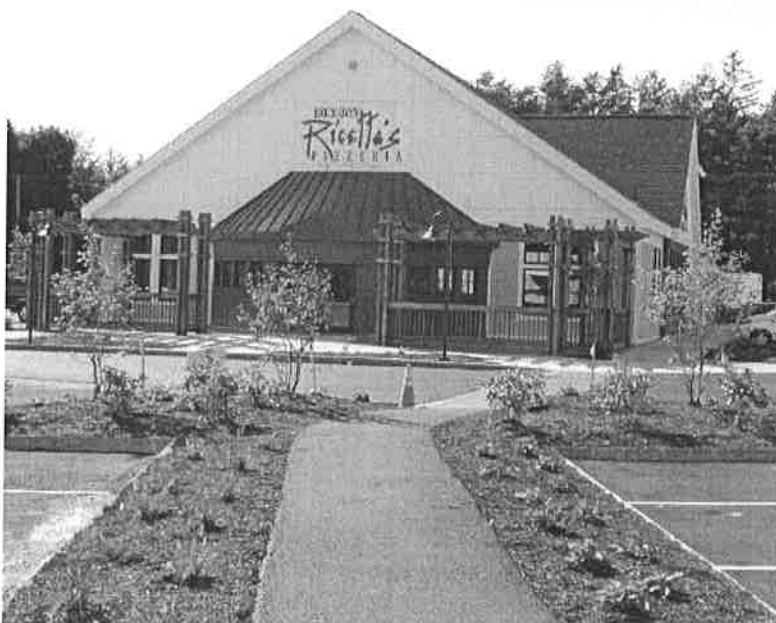
An internal walkway oriented toward the main entry of a restaurant in a multiple building development. The planting strips with ornamental grasses and perennials separate the pathway from overhanging bumpers.
