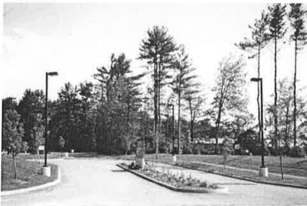
This curbed, landscaped island divides entering and exiting traffic. The identification sign is located away from the intersection to avoid interfering with the motorists' line of sight.
