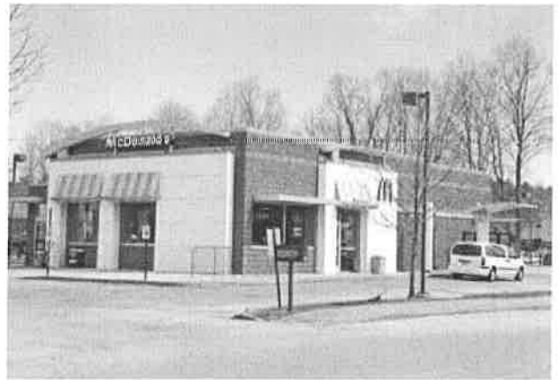
A national franchise that has been designed with a 'kit of parts' approach. The result is a box with applied facade features that has no reference to New England design, and would not meet these design guidelines.
