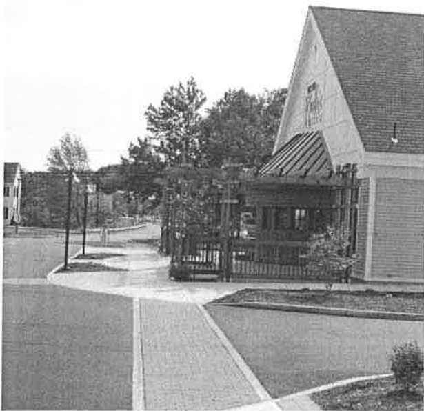
Concrete pavers create a permanent crosswalk that affords good visibility and contrasting surface texture.
