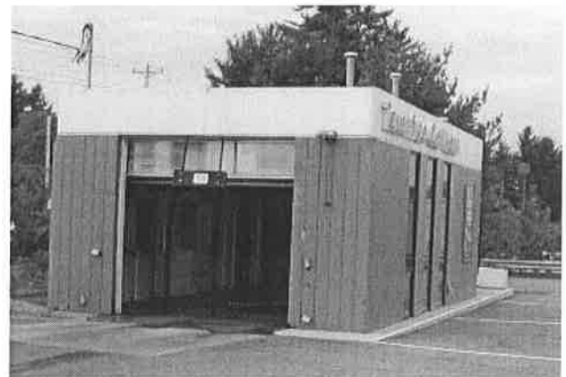
An accessory structure (a freestanding car-wash) that would not meet the design guidelines for form and materials.
