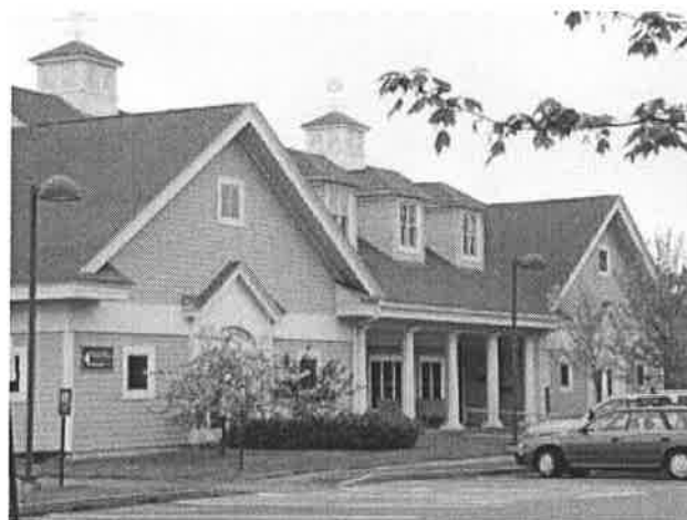
Examples of high quality contemporary Maine architecture -- a branch bank, a veterinarian's office, and a library - that have been designed to fit their unique sites.
