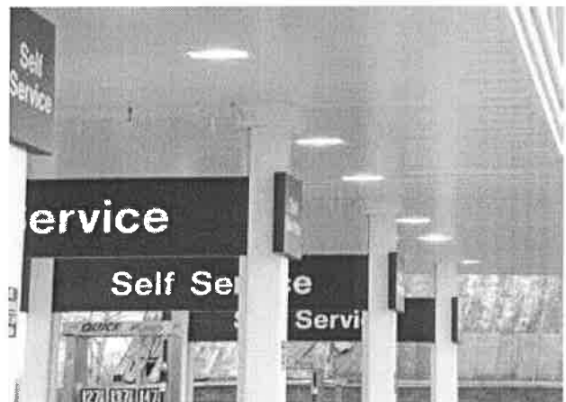
An example of dropped canopy fixture that spills light beyond the property line and causes potentially hazardous glare.
