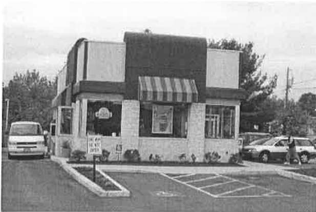
Corrugated plastic panels
