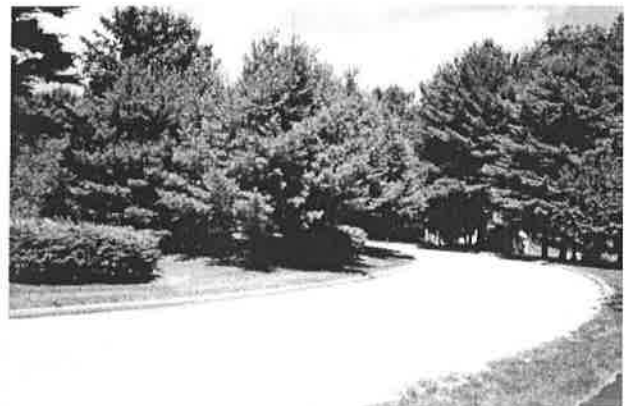
A 6-8' high earth berm, planted with evergreen trees and shrubs, creates an effective screen to separate an access drive from residential properties.
