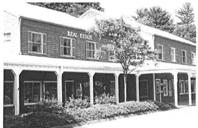
Covered walkways add a shadow line which can reduce the scale of a long building and unify its facade.
