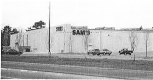
Painted concrete block
