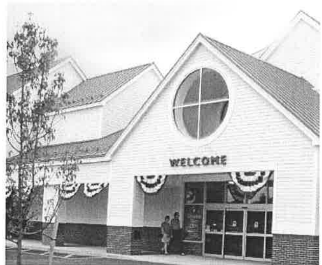
The main entrance to this grocery store is emphasized by the circular window. Brick banding gives visual support to the building while providing protection from snowplows.
