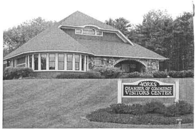
An unusual roofline derived from the shingle style makes a distinctive profile while maintaining a New England aesthetic.
