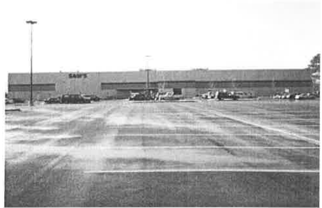
Landscaped islands should have been used here to provide scale, reinforce internal circulation routes, and lead pedestrians to the entrance.
