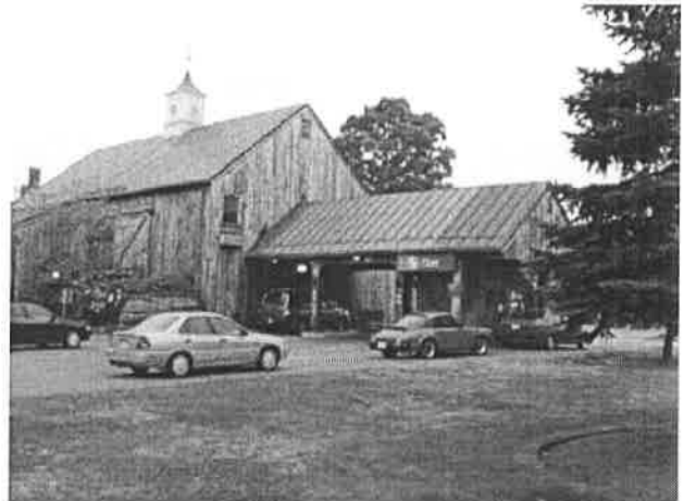
The design of this drive-through bank continues the theme of adaptive re-use and traditional materials.
