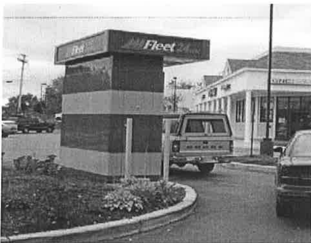
This ATM machine does not relate in form, color, or materials of the adjacent building.
