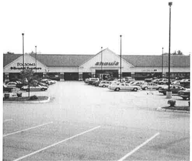
These lighting fixtures are taller than the main building and out of scale with the site.
