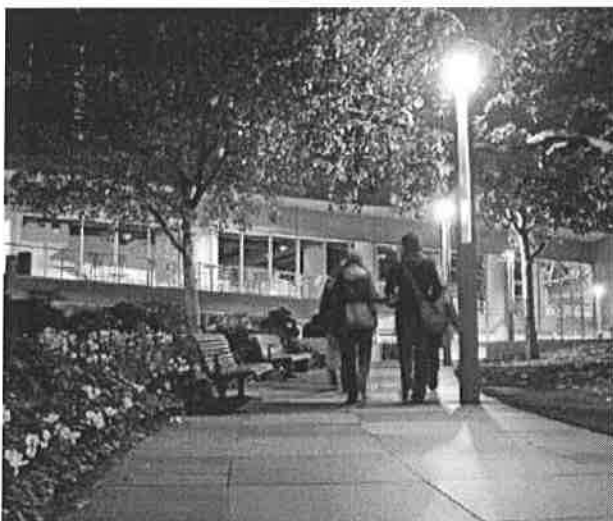
The glare from this unshielded walkway light may make it difficult to recognize faces of oncoming pedestrians.
