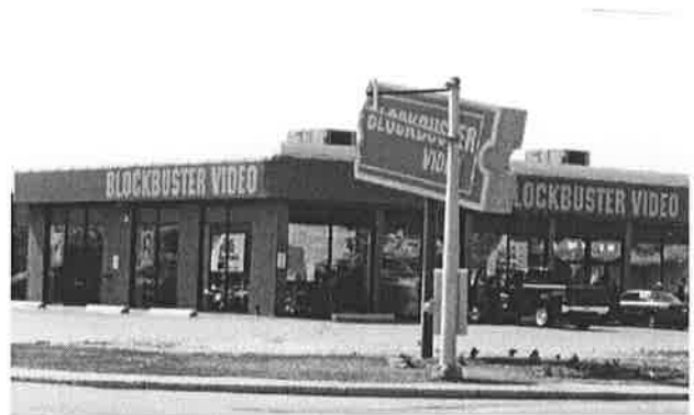
Advertising features, such as this overscaled ticket and internally lit band of color behind the facade sign, may be unnecessarily distracting and contribute to clutter.
