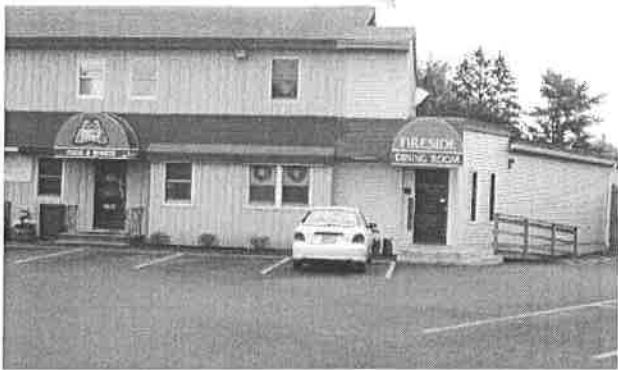
The addition to this restaurant does not relate to the form or building materials of the existing structure.
