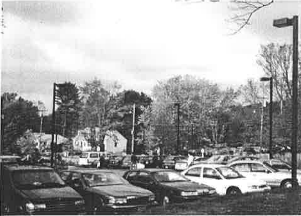
Lighting placed at the circumference of this parking lot blends into the surrounding trees, reducing its visibility during the day.
