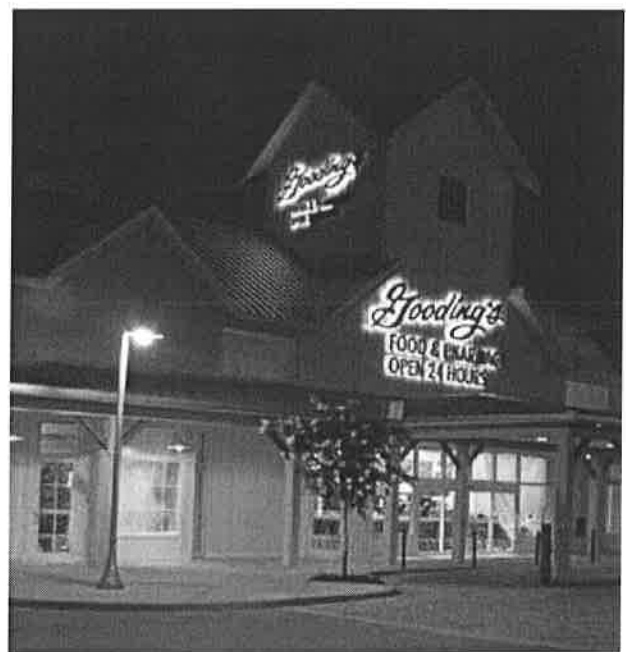
The lighting plan for this commercial building considers both security and visual appeal for motorists and pedestrians.
