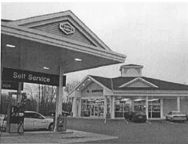
The gas station canopy has been designed to complement the main building. The town strongly encourages the use of attached canopies, especially in service stations that are being retrofitted.
