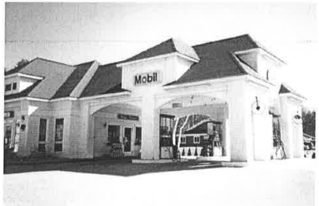
This service station canopy is designed to be an extension of the building. The columns, roofline, dormers, and signage contribute to a sense of continuity in the architecture.
