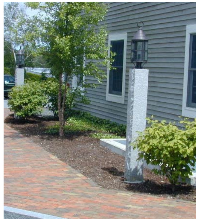
A light fixture that complements the surrounding architecture and site through the use of similar materials and appropriate scale.
