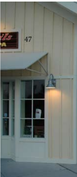
The wall-mounted light fixture on the right appears too small in relation to the height and scale of this large retail store. A proper installation is seen in the left photo.
