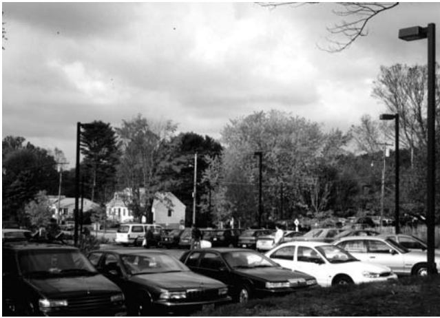
Lighting placed at the circumference of this parking lot blends into the surrounding trees, reducing its visibility during the day.
