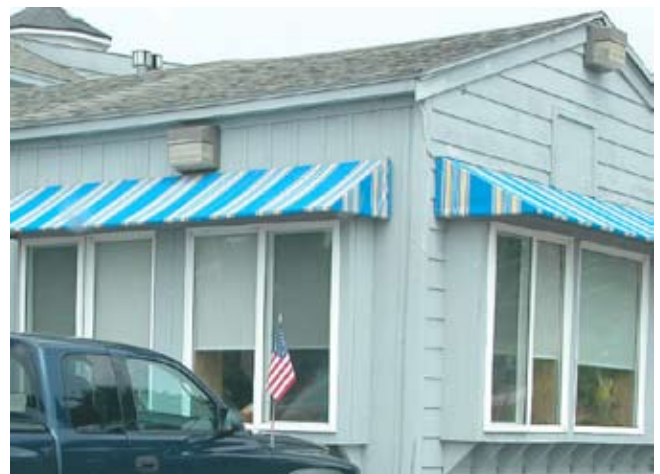
Unshielded facade-mounted lights are not allowed because they cause glare and spill light onto adjacent properties.
