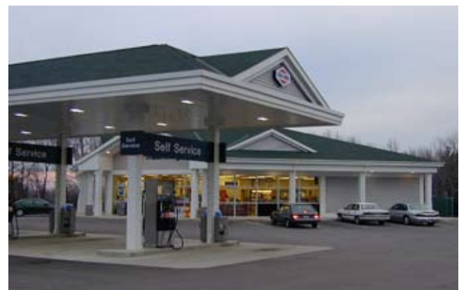
Lighting should be considered as an integral part of the canopy design. These canopy fixtures are recessed so the light source is not visible and do not create 'hot spots' that are distracting to the passing motorist.
