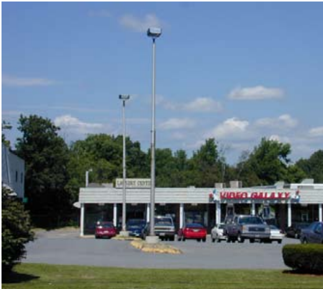
Spotlight fixtures should be avoided since they are difficult to aim and may cause spillover onto adjacent properties.
