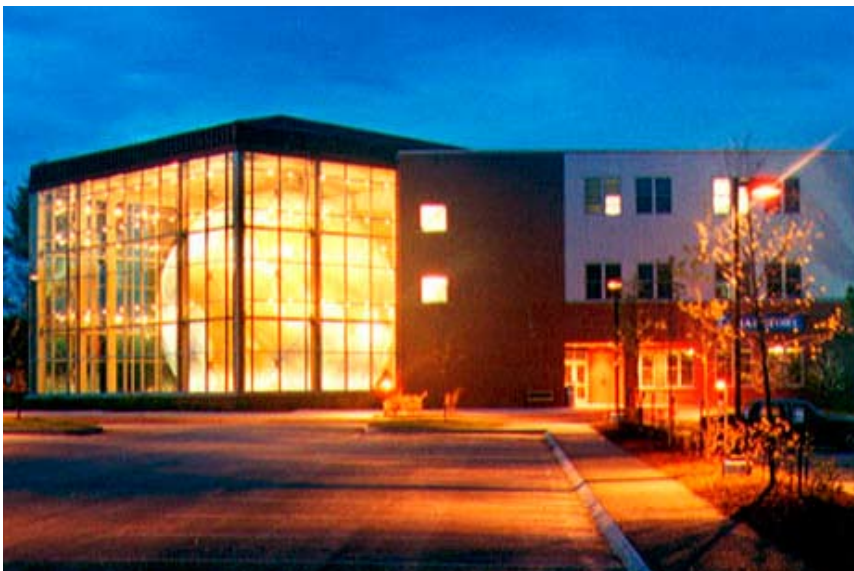
This parking lot lighting illuminates the walkway and emphasizes the route to the front door.
