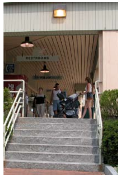
Unshielded wall-pac lighting can cause dangerous glare and make it difficult to see the stairway.
