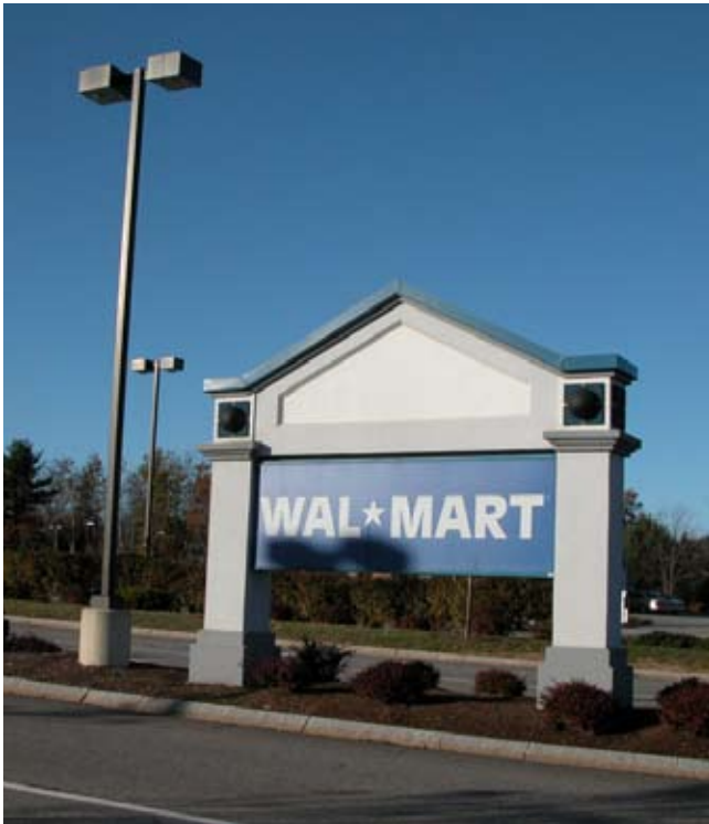
Simple 'shoe-box' fixtures mounted on square poles provide a clean look that complements the site.
