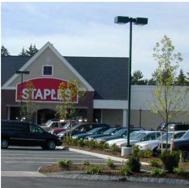
These light fixtures have been coordinated with the planting plan to avoid problems as the trees mature. Slightly raised bases protect the poles from plow damage.
