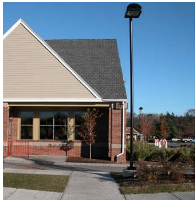
A cut-off fixture that complements the simple line of this commercial building. The fixture is mounted on an 18-foot pole on a one-foot base for an effective height of 19 feet.
