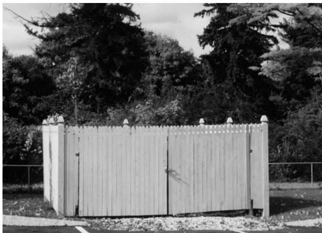
A typical trash enclosure. Its appearance could be improved by plantings along its sides, detailing to match nearby buildings, reinforcing the gates, and staining a dark color.
