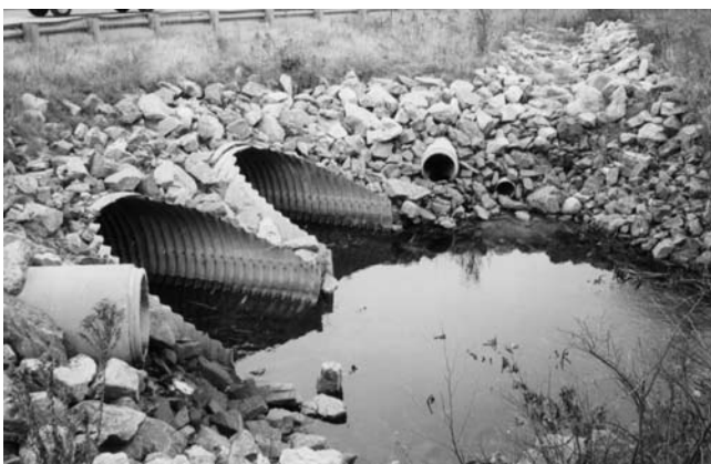
Rip-rap is often necessary to control erosion and stabilize slopes. In highly visible areas, a more refined appearance – accomplished through the use of handplaced stone and/or ground cover – is necessary to avoid situations such as this.
