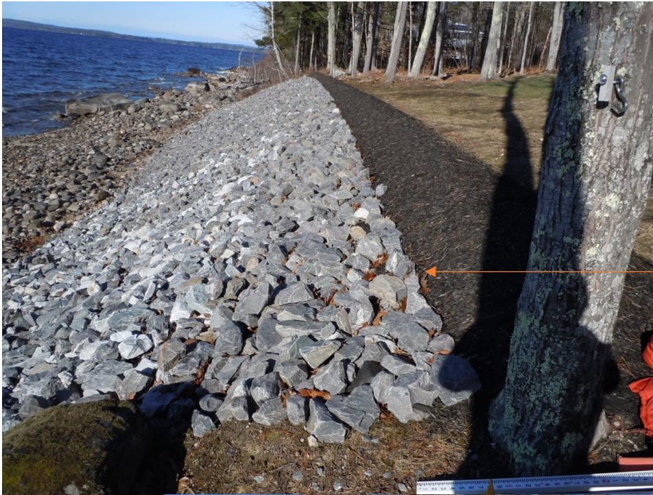
Post Construction Riprap
