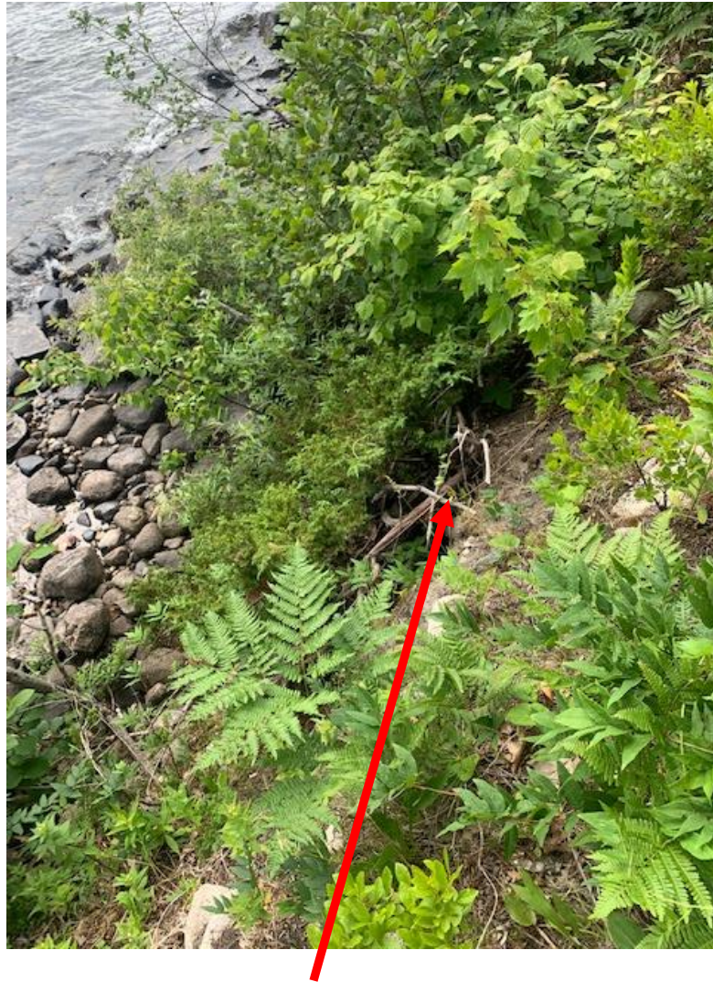
Soil erosion present beneath vegetation foliage
