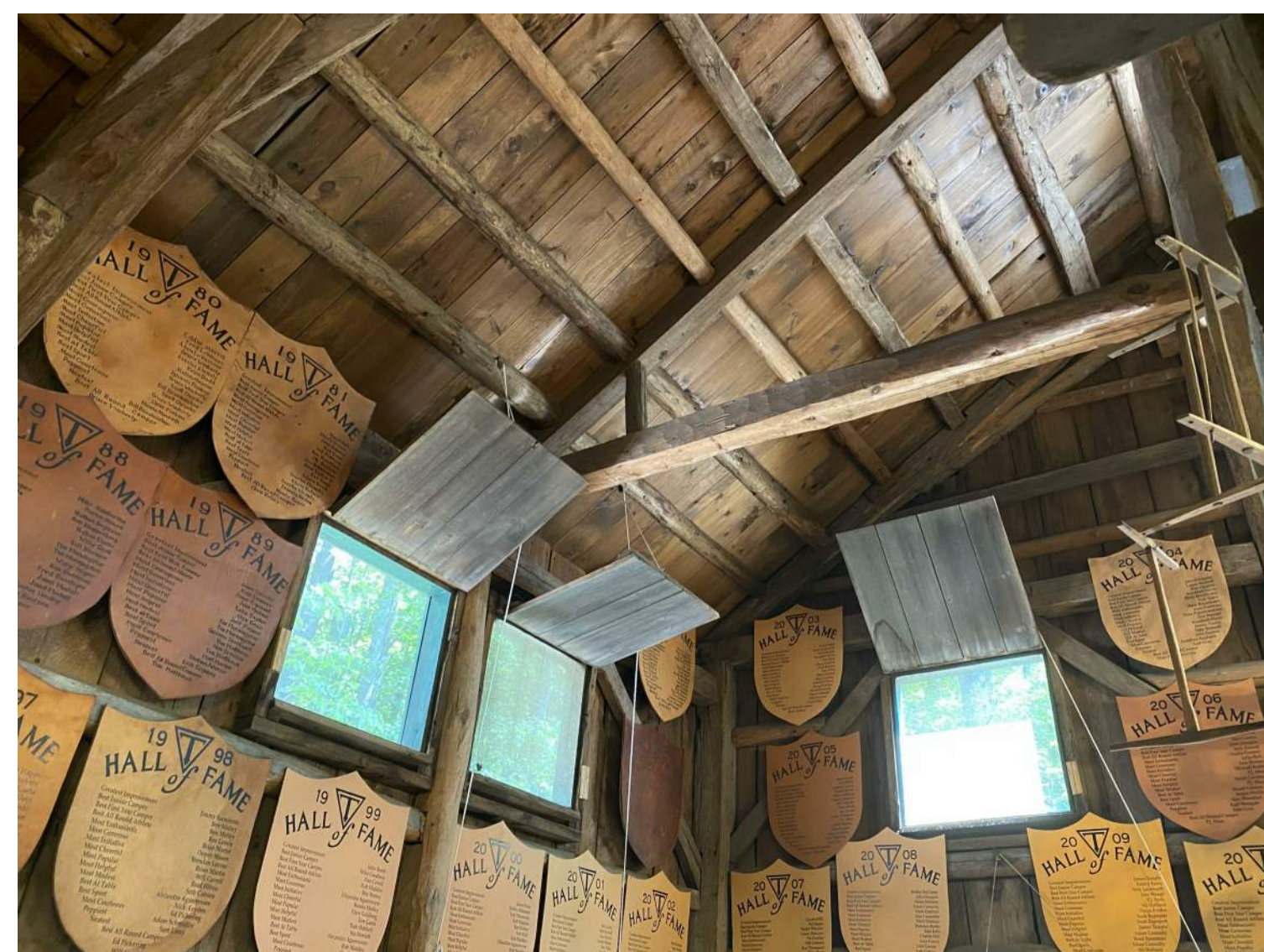
REFERENCE IMAGE OF EXISTING CONDITION
