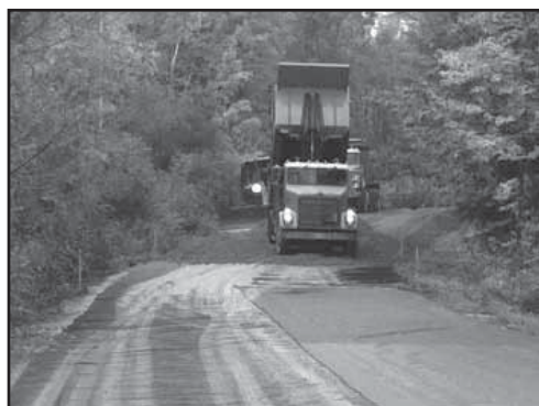
Spreading base gravel over geo textile.
