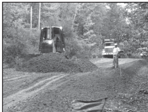
P&K spreading sand and gravel over geo textile.
