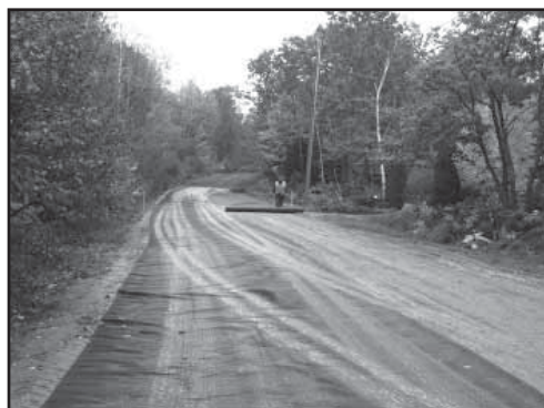
Scott Picavet laying down geo textile on Tenny Hill Road.
