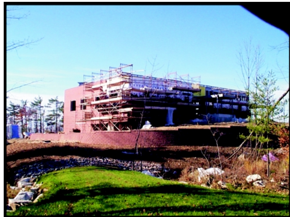
View of the new school from the catch basin.
