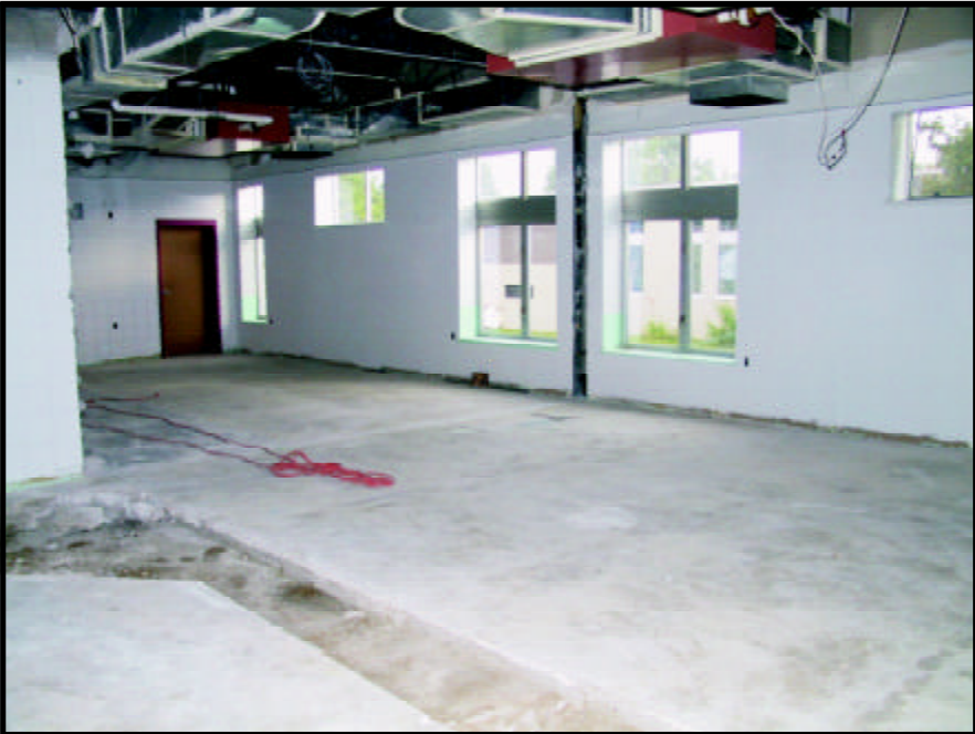
Two rooms becoming one of our two new Science Labs! One wall has been taken down, and the floor has been cut for new plumbing.
