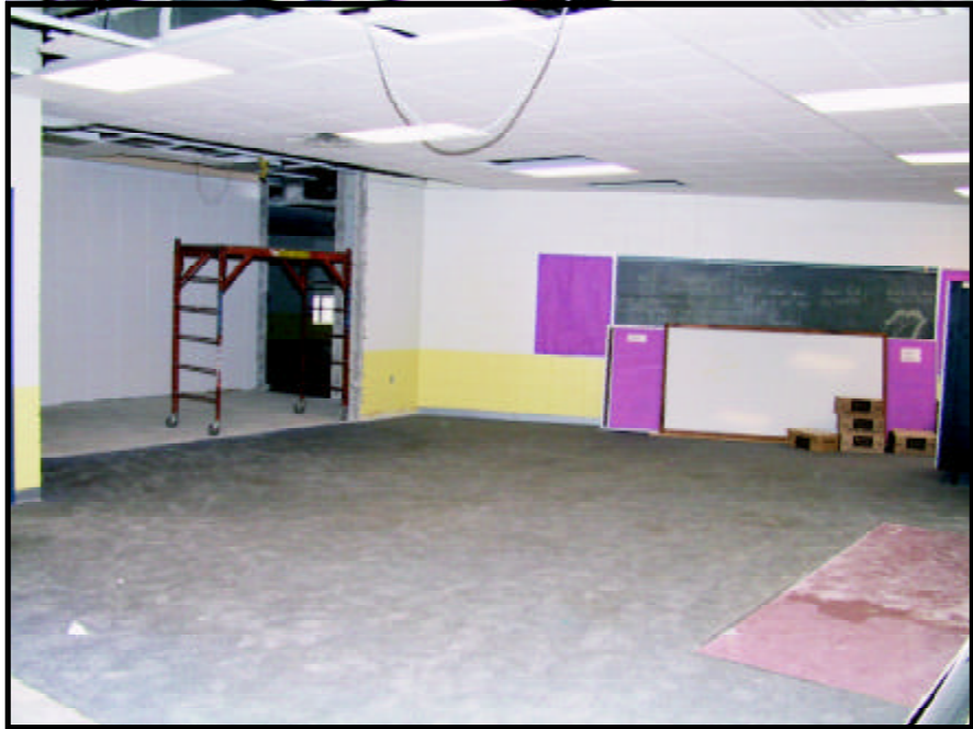
Looking through an area where two walls are being replaced by new walls with lockers inserted into them. In the background you can also see where new ADA doorways are being built.
