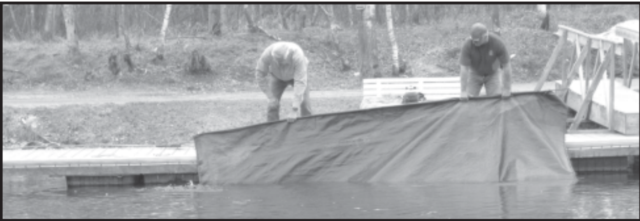
Port Harbor Marina Staff Laying Benthic Tarps to Control Milfoil
