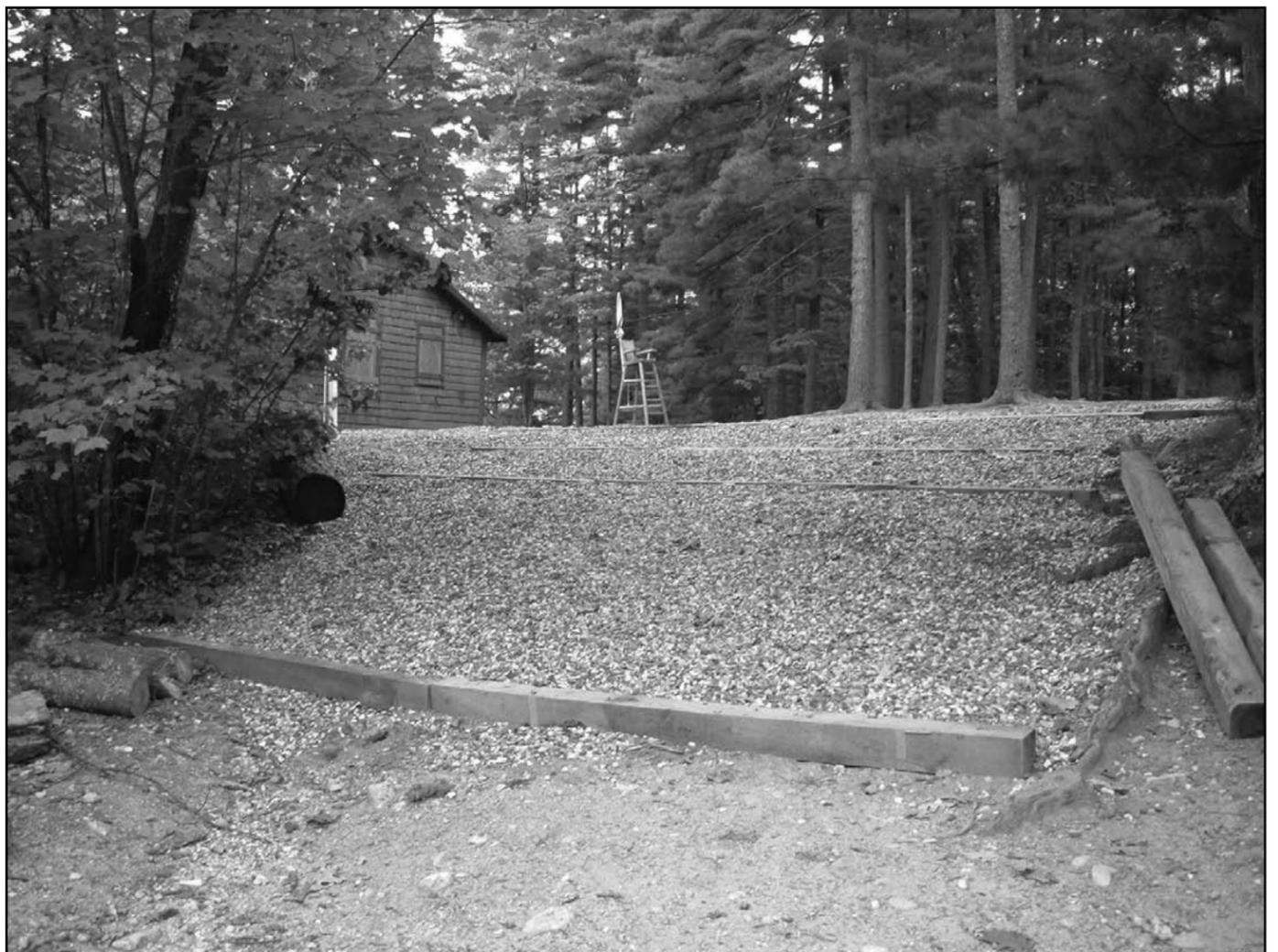
*AFTER: 60'x4'x4' Rock-filled infiltration trench at edge of parking area, infiltration steps on path.*
