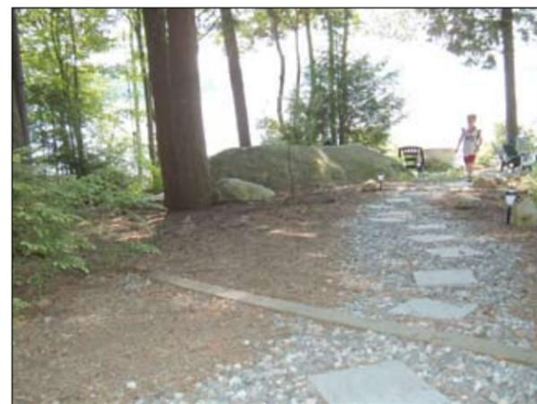
The Watsons installed a crushed stone path with waterbars to divert water into vegetation; spread erosion control mulch; and planted blueberries on both sides of the path.
