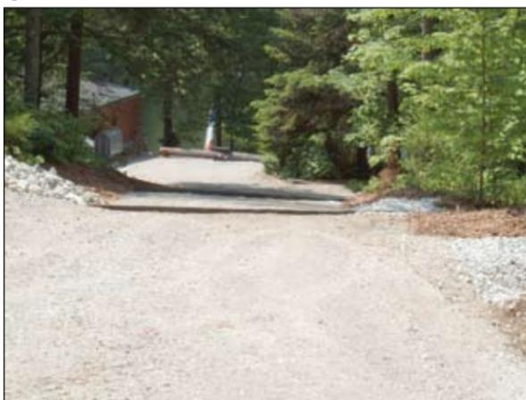
Rubber blade diverters direct water into rock-lined outlets
